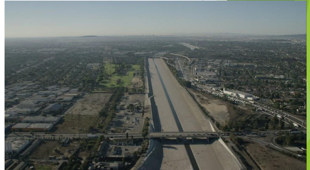
Aerial image of I-710/I-105 interchange-Lynwood, CA
